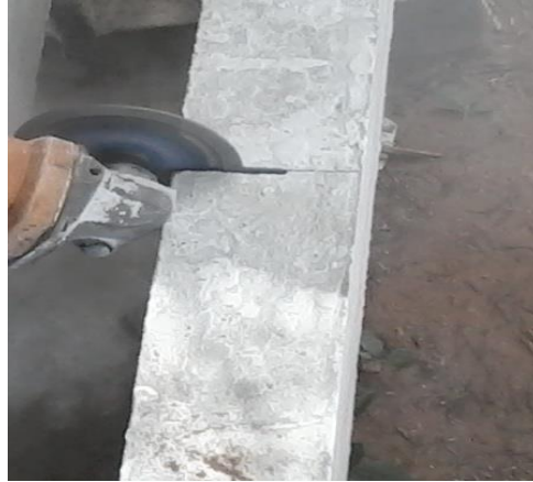
FIGURE 3.1 cutting beam with marble cutter.
